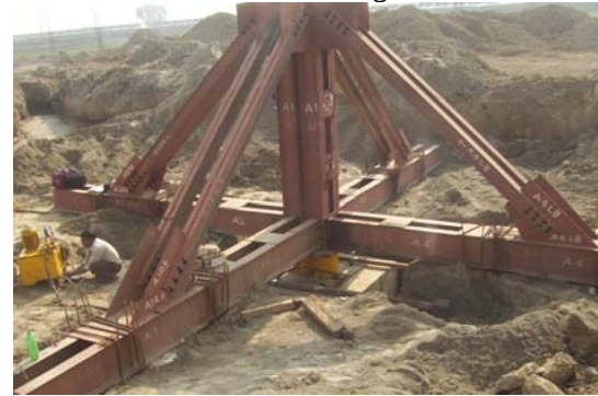
Fig. 3. Set-up for footing load test
