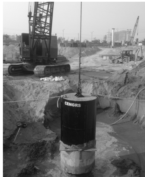
Fig. 7. Hammer Impact on Pile
