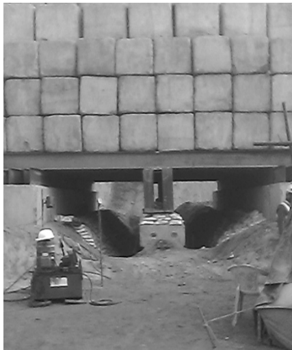
Fig. 2: Load Test Set-up
