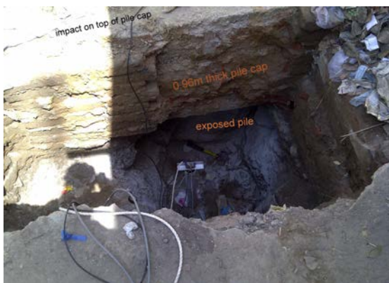
Fig. 4 Parallel seismic test set-up
