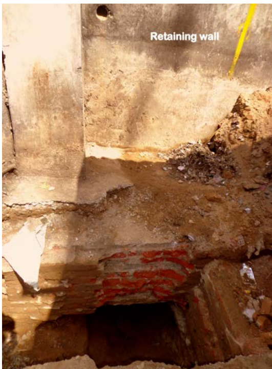
Fig. 2 Trial pit showing exposed pile
