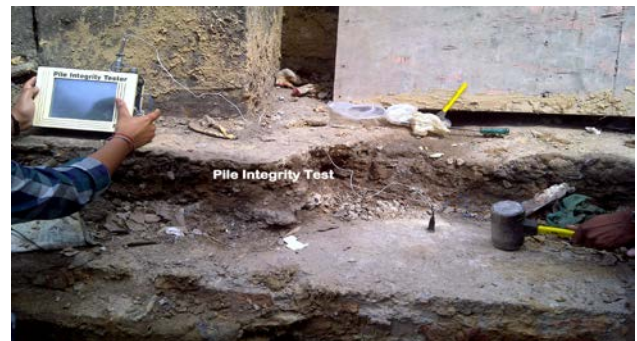
Fig. 6 Sonic echo response test in progress
