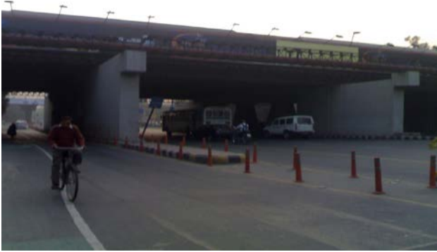
Fig. 1 A view of the bridge
