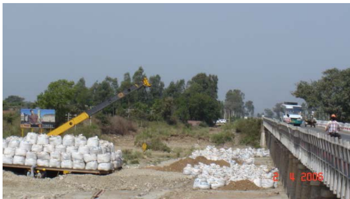
Fig.8: Footing Load test in progress
