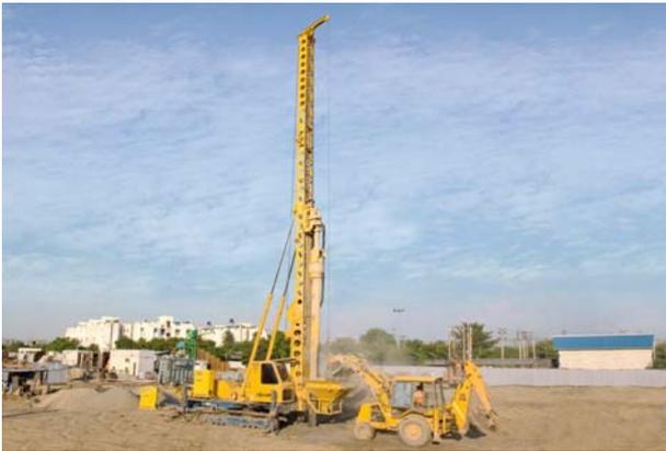
Fig. 6 : Vibro-replacement in progress
