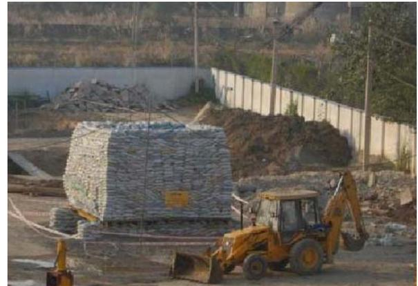
Fig.8 : Load Test on Stone column
