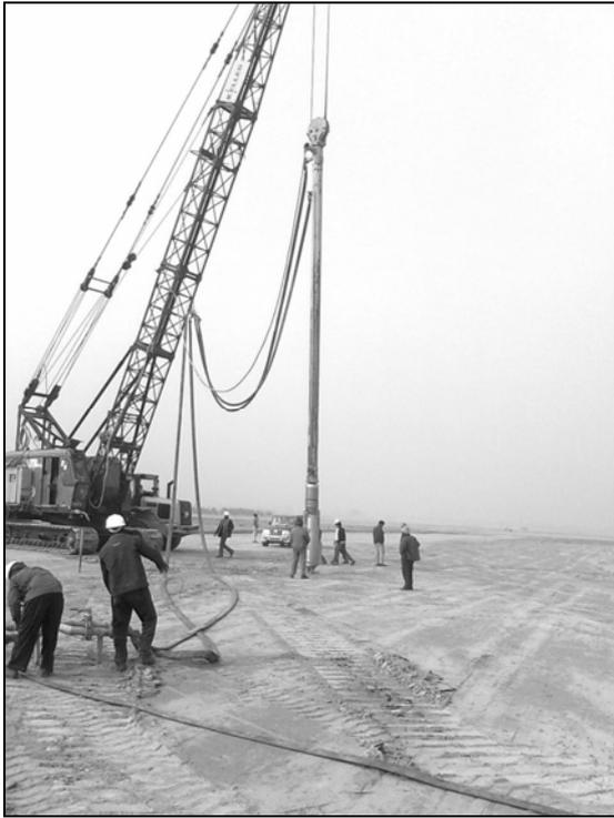
Fig. 5 Vibro-compaction in progress
