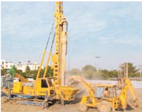
Fig. 7: Vibro-Replacement in progress
