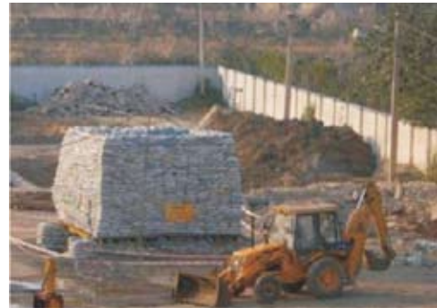
Fig. 9: Load Test on Stone column
