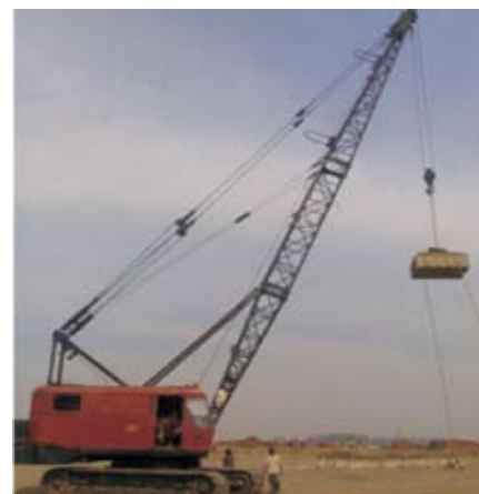
Fig. 14: Dynamic Compaction in progress on site
